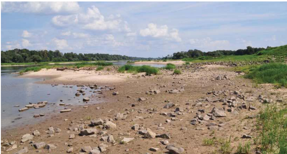
Fig. 18. An example of groyne destruction after flooding, the Elbe River near Dessau in Germany, August 2013. The rip-rap of the groyne was washed downstream and deposited on the sand inside the groyne field. An apparent breach is visible on the right side of the groyne as well as a sand bar deposited at the separation zone in the middle of the groyne (the view is upstream of the river from the left bank)
